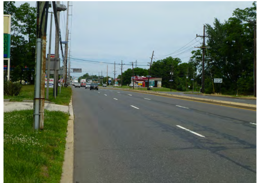
Figure 17: CR 541 at Connecticut Drive
